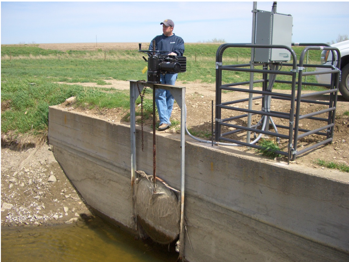
Figure 2. Project staff testing the functionality of a newly installed automated head gate on the Sorenson Lateral prior to the 2007 irrigation season.
